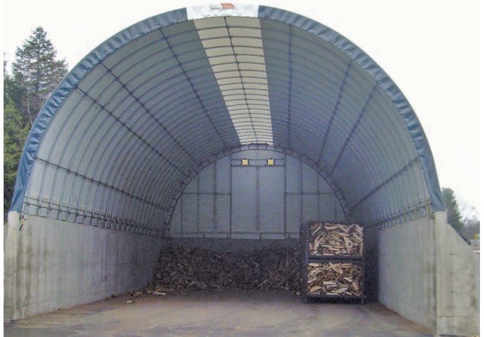
ClearSpan storage building stores and protects kiln dried firewood. Treehugger Farms provides quality kiln dried and debarked firewood for its customers.
